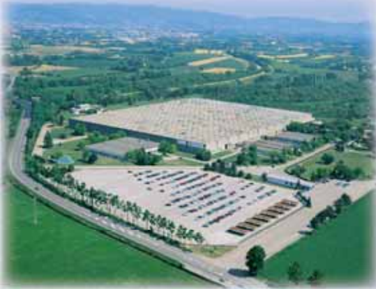
Manufacturing Plant Arzignano - Italy
