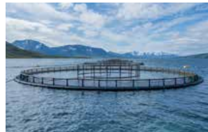
Most plastic cages are moored in a grid system and include sinker tube, centersupport stand, feed system/ barge, cameras and sensors.
