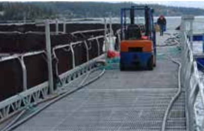
Fully integrated and extra wide non-slip walkways, net supports and floats with self-draining top.
