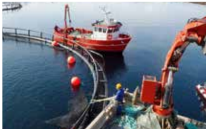
Polarcirkel EcoNet being installed by use of cranes and skilled farm technicians.
