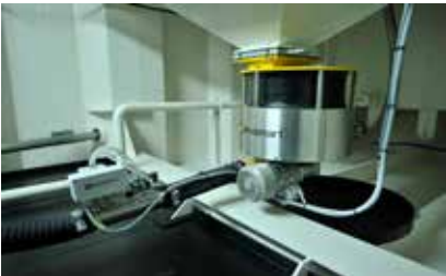
The Feed Doser Valves have capacities from 0,6kg/min. up to 192kg/min.
