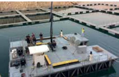
Local deck installation The modules are transported to the location in parts and installed by experienced Wavemaster staff.
