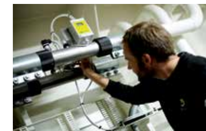
The Air Control unit is installed between the Air Cooler and Feed Doser Valve.
