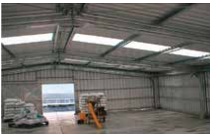
Hot dip galvanized construction All structural steel components are hot dipped galvanized after manufacture. This has proven to be the most effective and durable coating for use on fish farming structures.
