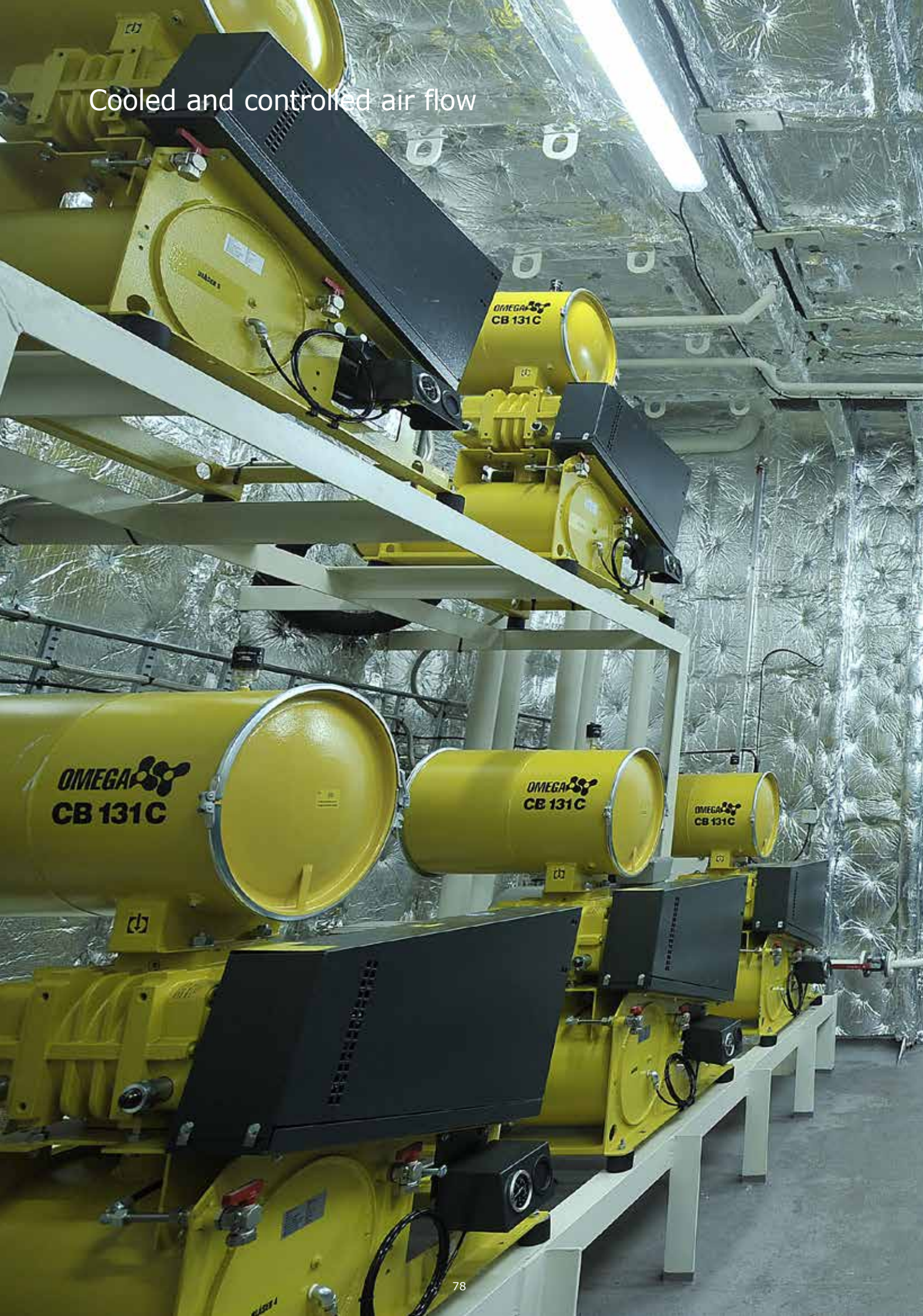
Sound protected machine room with Feed Blowers and generators.
