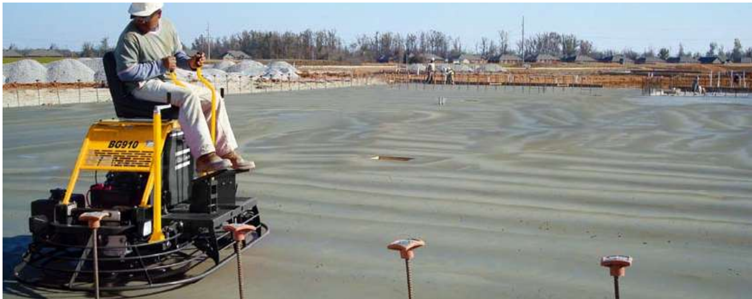
A thumb button on the steering lever controls the water spray system on BG740 and BG910.
