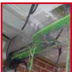
False floor and false ceilings
