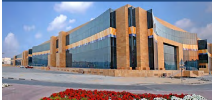
Financial Square Building, Qatar
