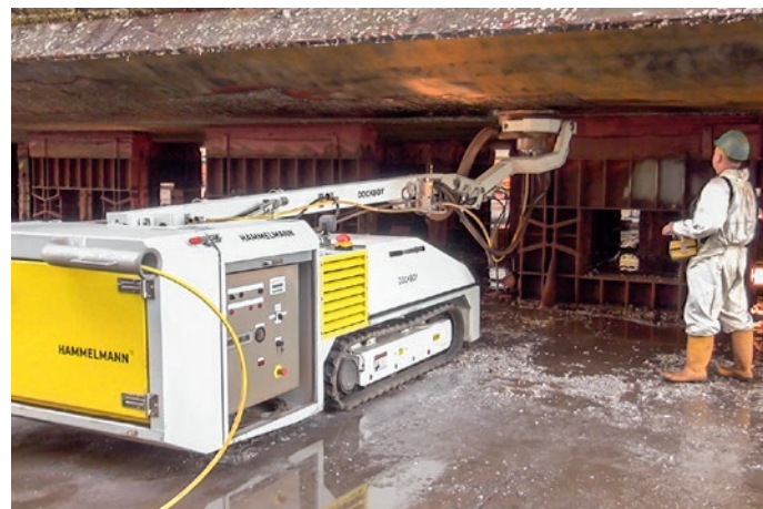
Dockboy - surface preparation on ship hull bottoms
