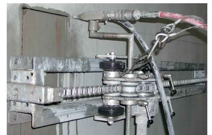
Abrasive cutting injectors and handling equipment
