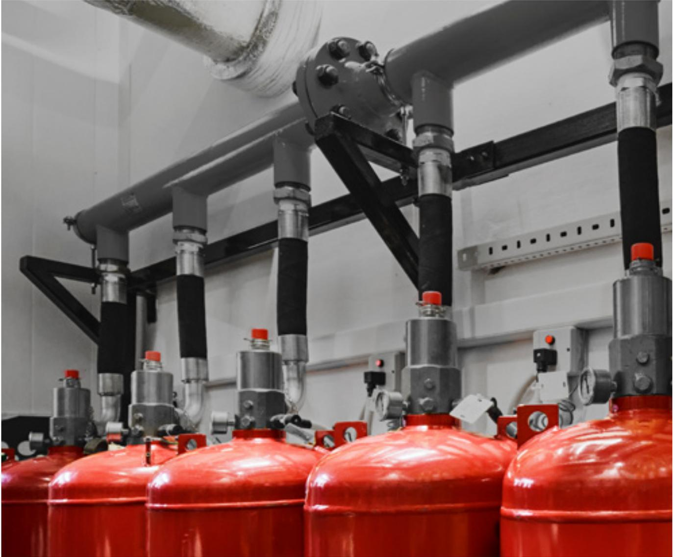
LIFECO5112 system cylinder valve assemblies are Equipped with pressure differential high flow rate valves in in order to meet the rapid discharge time of 10 seconds as specified in NFPA 2001. LIFECO5112 has a wide filling range from 20 lbs to 1200 lbs allowing for head valve outlets ranging from 1" to 4". LIFECO5112 cylinder head valves have been designed to be actuated electrically, pneumatically or mechanically, to make it suitable for different designs application
