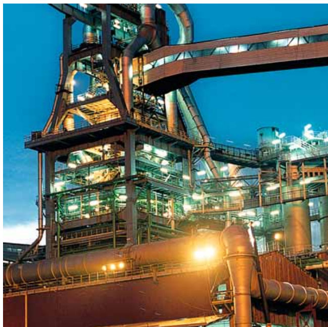
Industrial application: Refinery
