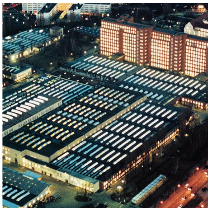
Switchgear Factory, Berlin, Germany
