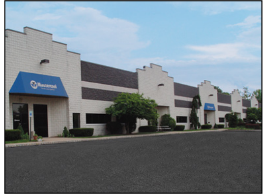
European Sales Office and Warehouse
