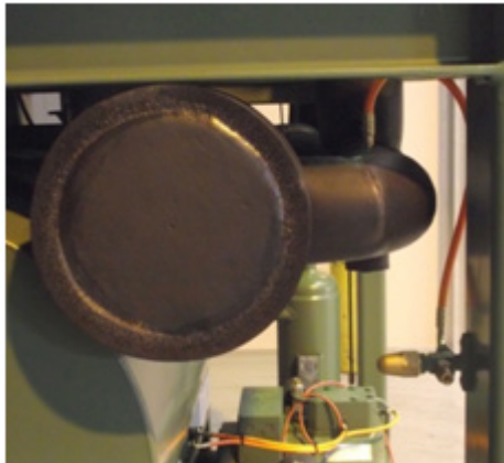
Figure 18A - Liquid Line Drier
