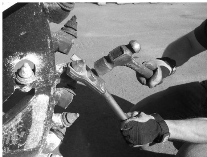
New Pick Installation
