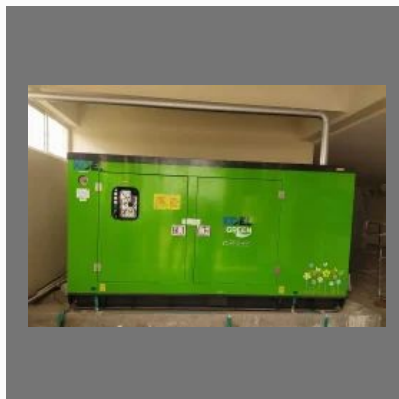
15 kVA KOEL by Kirloskar Diesel Generator
