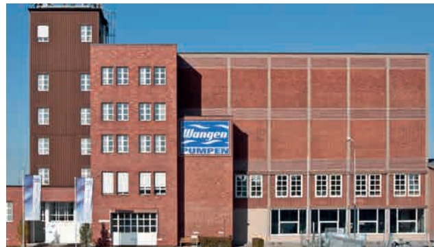
Headquarters building in Wangen, Germany
